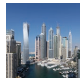
DUBAI Saving energy in air conditioning systems
